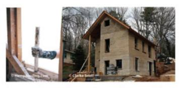
Hempcrete can be cast maually around a timber frame using a shuttering system. This creates a uniform evenlope to the structure which achieves a high standard of insulation and consequent low energy consumption with additional health benefits especially humidity regulation.
