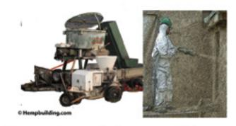
Hempcrete can also be sprayed intp position more quickly and produces a superior material that sets and dries out in less time
